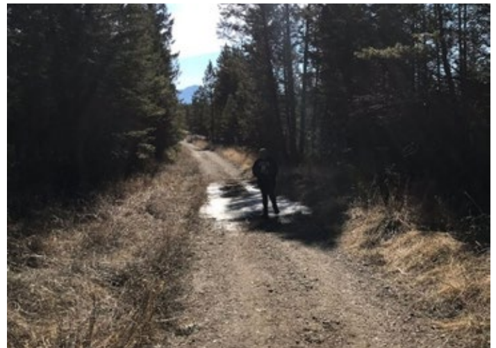
Figure 37 Minor Cupping and Berming Visible on the Old Coach Road Trail (Photo Credit: Lora Cook, AllTrails)
