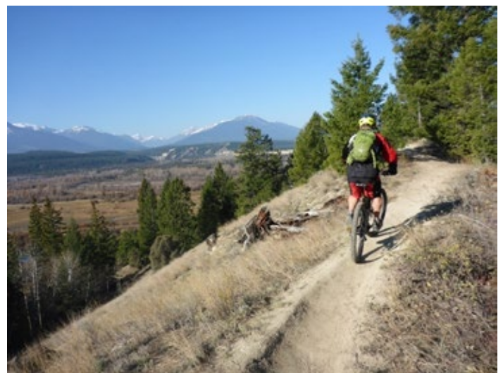
Figure 38 Cupping and berming (foreground) on Deja View Trail (Photo credit: Singletracks.com)
