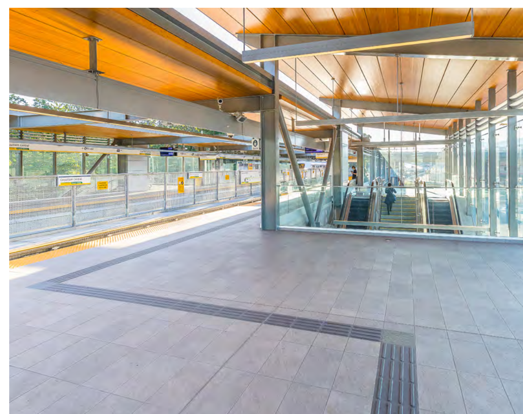
Example of tactile wayfinding tile in contrasting colour at the platform
