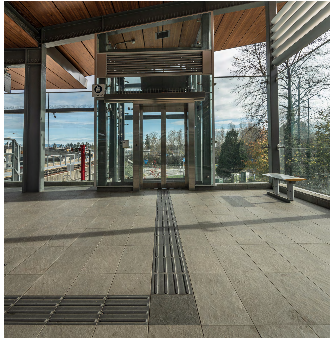
Example of tactile wayfinding tile in contrasting colour, leading to key destination
