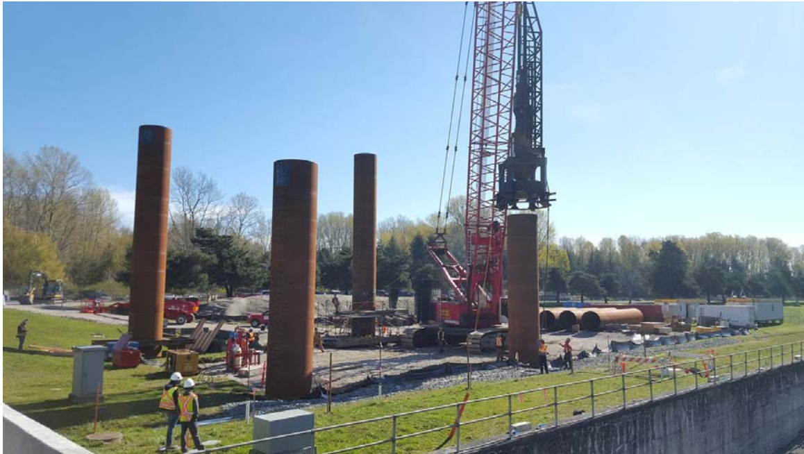
Pile installation
