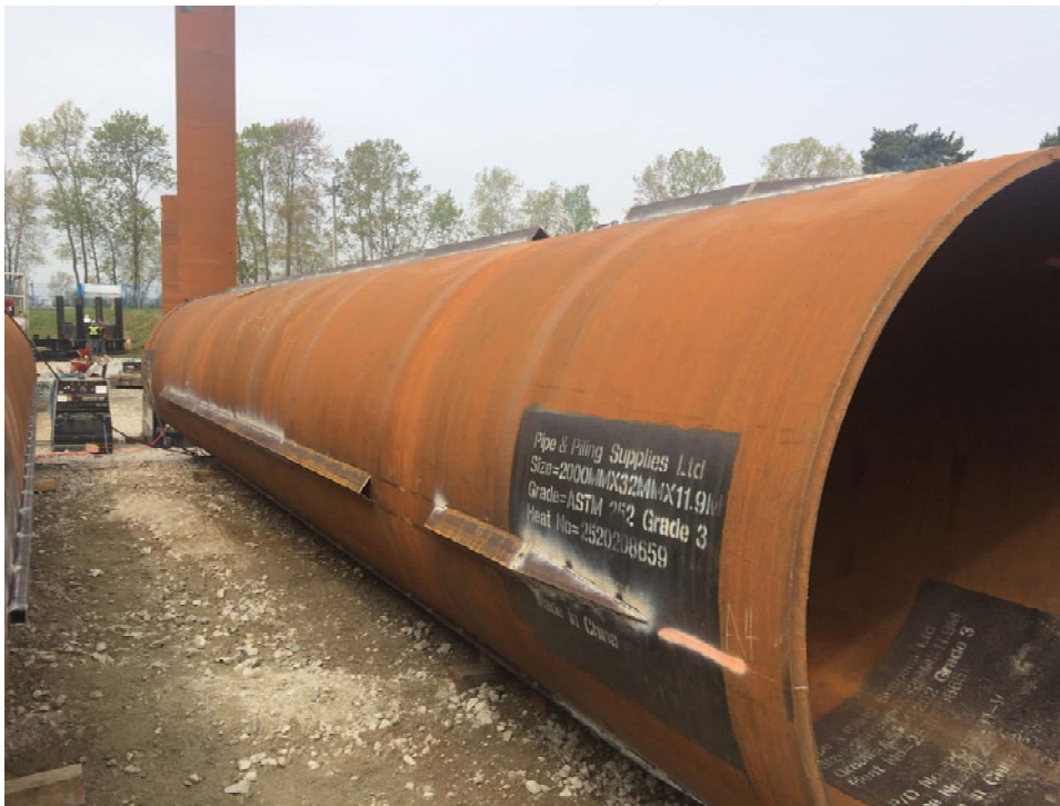
Test pile instrumentation protection
