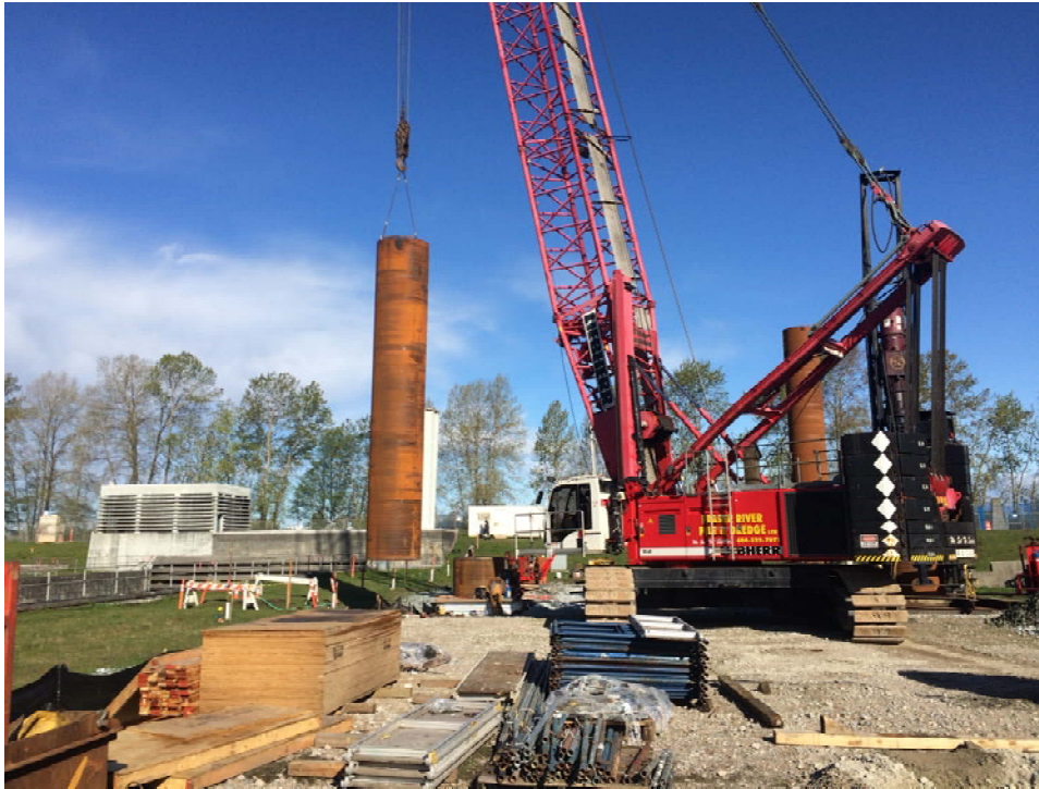
Hoisting pile for stacking
