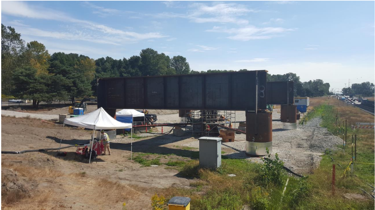
Instrumentation testing prior to static load test
