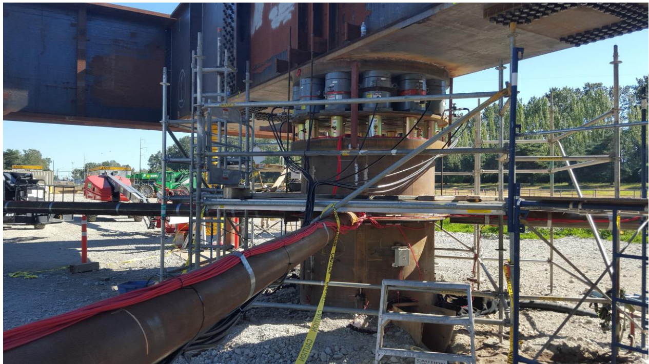
Setup for static load testing
