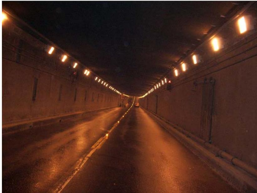
Figure 3 - Existing Tunnel Lighting
