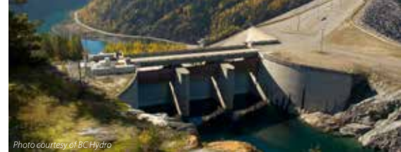
Photo courtesy of BC Hydro
