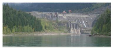
The minimum and maximum licensed levels for Revelstoke Reservoir are 554.7 metres (1,820 feet) and 573.0 metres (1,880 feet) respectively. At most times, Revelstoke Reservoir levels are maintained at or above 571.5 metres (1,875 feet).
